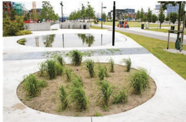
4.49 Open ponds and vegetation gardens in parks are used to purify stormwater before it flows to the sea.
