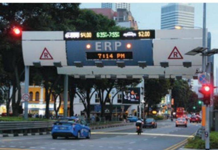
3.38 Electronic Road Pricing (ERP) operates in the CBD of Singapore to regulate traffic congestion, with toll prices for entry varying according to congestion levels at different times of the day.
