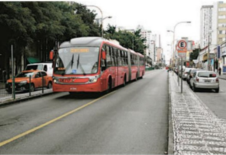
3.42 A two-way dedicated bus lane runs through the middle of a two-way central street in the trinary road system in Curitiba.
