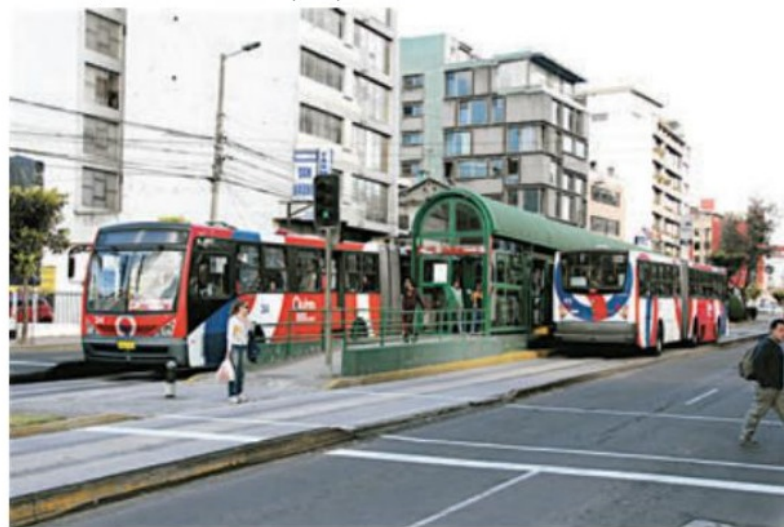
2.33 Transport infrastructure in Quito, Ecuador, has received substantial investment. Modelled on the system used in Curitiba, Brazil, separate bus lanes have been built on main roads, with covered bus stops positioned for rapid boarding.
