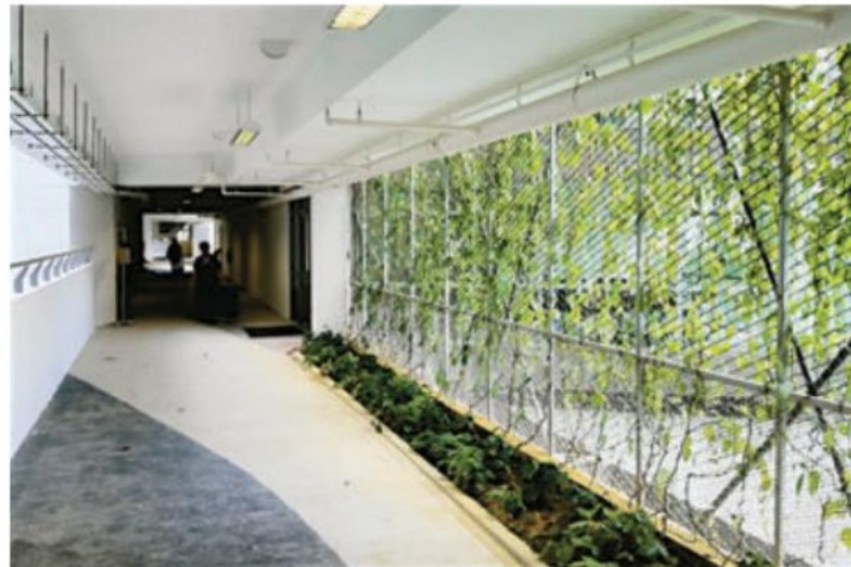
4.42 This elevated bridge joining two buildings in a school in Singapore has a 'green wall' which reduces the heat load in the building's interior in the hot, tropical climate.
