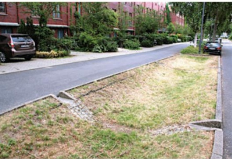
4.74 A close view of roadside bio-swale shows the open channels that allow water to drain from the road into the swale.
