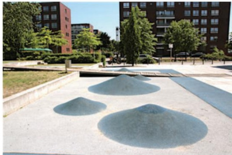
4.72 Porous surfacing in Rummelsburg that allows water to infiltrate into the soil.
