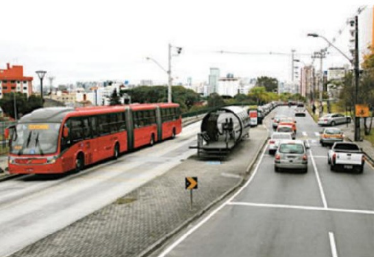
3.44 A two-way bus lane runs along the side of a one-way road for cars in suburban Curitiba.
