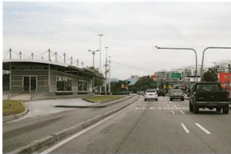
4.13 Avenida das Américas is one of the first roads in Rio de Janeiro to have its transport infrastructure upgrade. The road has been widened to relieve congestion, and separate bus lanes have been constructed so public transport is not delayed by traffic jams. The building to the left of the bus lane is the Interlagos bus interchange station.
