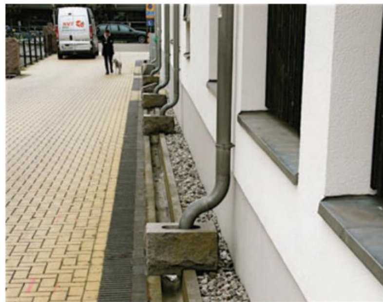
4.50 Drainage pipes and open channels in Western Harbour.
