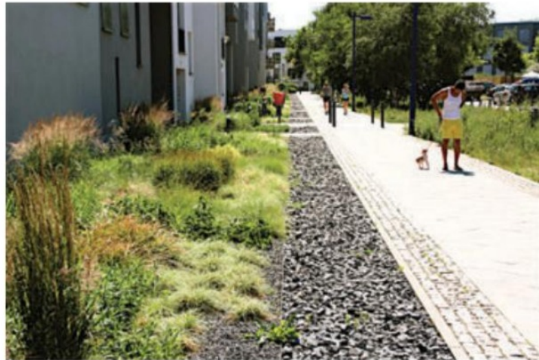
4.76 New housing on the Stralau Peninsula is lined with gardens of rainfall-absorbing plants and porous gravel that allows infiltration of rainwater.
